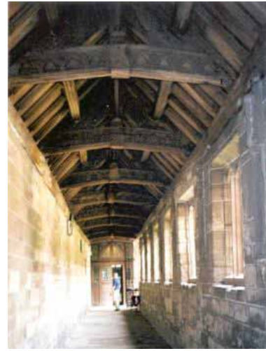
Figure 54 The passage into the Vicar's Choral showing the fine hammer-beam roof.
