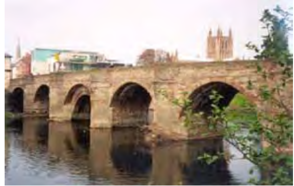
Figure 2. The Wye Bridge from the west, south bank.
