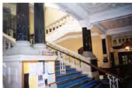
Figure 34. Entrance hall to the town hall showing dark pillars of the so-called 'Otta Phyllite' from Norway, which is a dark larvikite with
