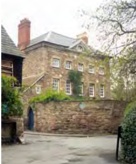
Figure 44. Harley House, a Georgian Building in local "old red sandstone", with a roof of Welsh Slates.
