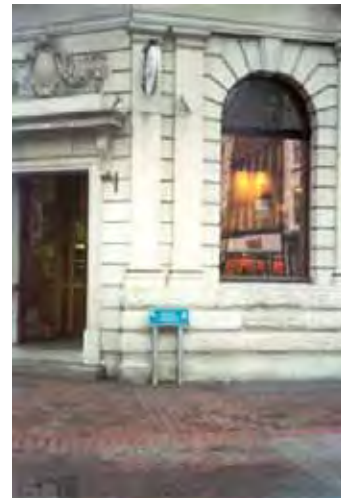
Figure 11. The HSBC Bank in Portland Limestone. Note the deliberate roughening of the lower four stone courses, a type of rustication. Rustication is also evident in bevelling of the smooth blocks above. The arch has a keystone.
