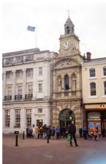
Figure 20. Façade of Butter Market in High Town showing the striped architectural effect achieved by alternating smooth (light) and rusticated (dark) limestone blocks.
