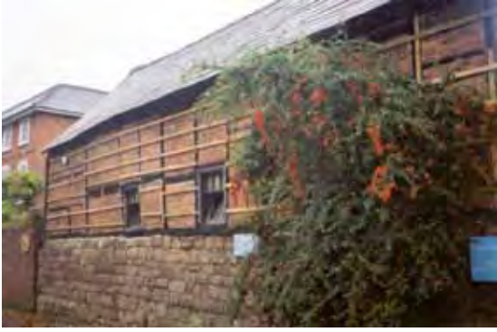
Figure 43. The 'Cathedral Barn'; a mediaeval 'hall'; stone in the lower part and timber framework with red brick panels above.
