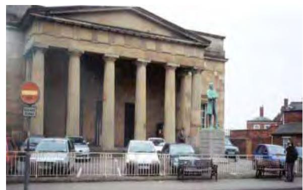
Figure 30. The classical façade of the Shire Hall faced with light brown sandstone ashlar. Note the bronze statue of Sir George Cornwallis-Lewis to the right.
