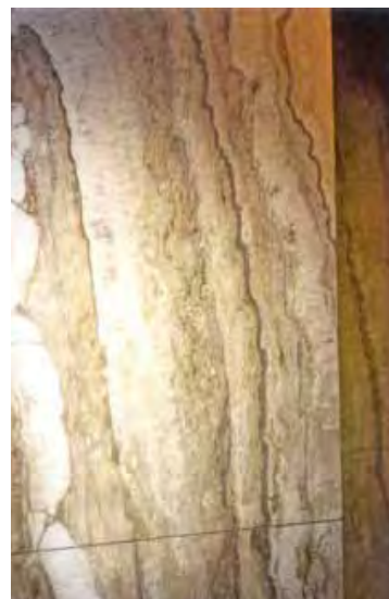
Figure 19. Cladding on the front of MacDonald's, travertine with the banding vertically arranged on the shop facing.
