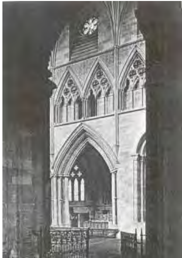
Figure 50. East wall of the North Transept with decorated gothic architecture: the dark pillars are of Purbeck 'Marble'.
