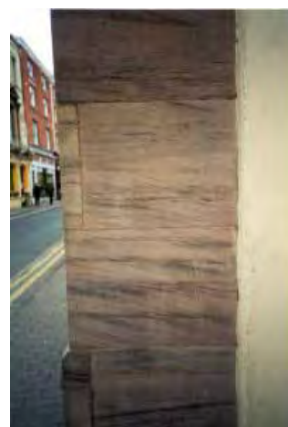
Figure 12. Cladding of sandstone in the façade of Primark in Widemarsh Street. This displays cross-bedding produced by water currents: it ranges from quite large foresets to smaller, ripple-scale foresets.
