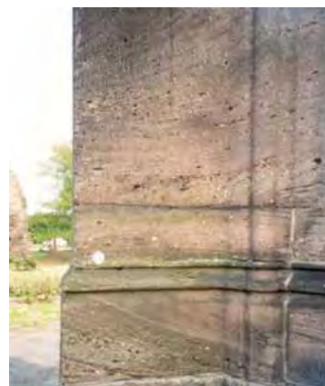
Figure 15. Close-up of Old Red Sandstone pebble beds with large-scale cross bedding foresets, used in the cross.
