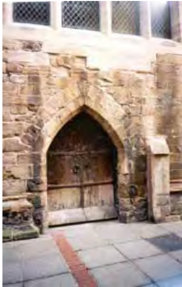
Figure 9. Transitional west doorway of the tower of All Saints Church, with pointed arch, in the same material, but with recent restoration above of the west window in sandstone from Derbyshire, now white but it will darken rapidly on exposure
