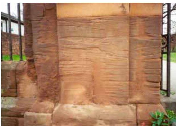
Figure 17. Close-up of the stonework of the arch, showing the 'hot' red colour of the Old Red Sandstone used, the cross bedding and the weathering produced by a century of exposure to city fumes. The sandstone displays channelling features, typical of fluvial (river) deposits. Now turn right and walk to the traffic lights at Blueschool Street. Note more sections of the city wall. Cross over and walk up the west side of Commercial Street opposite. Here we will see some interesting claddings.
