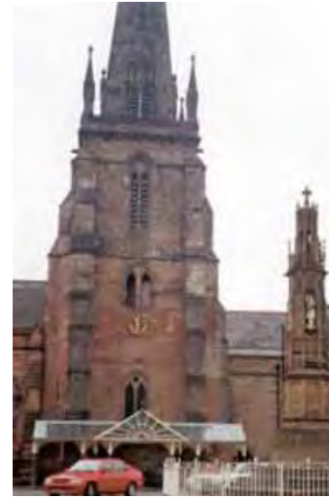
Figure 28. View of the tower and spire of St. Peter's Church. The upper part original stonework, the lower part restored. Note the war memorial on the right modelled on the mediaeval Eleanor Crosses.
