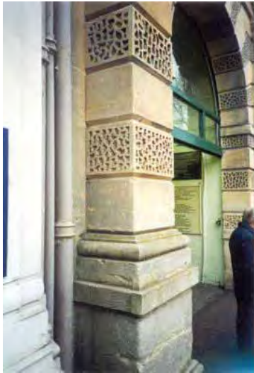
Figure 21. Close-up of the Butter Market stone blocks, which are very stained but could be Cotswold Limestone.
