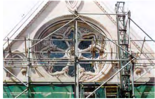
Figure 62. The east end of the Cathedral, rebuilt in sandstone from Derbyshire. This is white when installed, but weathers darker to match the local stone.
