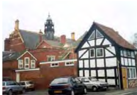
Figure 33. The brick and Welsh slate construction of the Town Halls seen from the rear, contrasting with the terracotta façade; and a small mediaeval lath and plaster building adjoining it in East Street.
