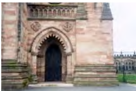
Figure 69. Part of the West Front, as it is now, in Hollington Stone.
