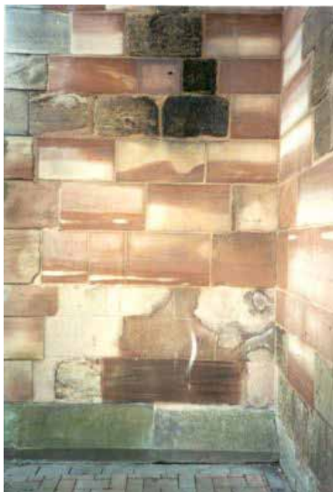
Figure 27. Restored walling with tightly-fitting ashlar blocks of smooth-faced Hollington Sandstone (Triassic "new red sandstone").
