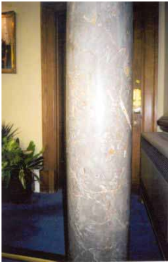
Figure 35. The pillars on the stairway in the entrance hall of the town hall, of a veined grey marble with red patches.
