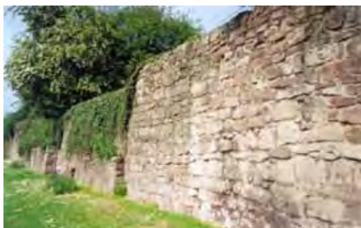
Figure 5. The city wall to the east of Victoria Street
