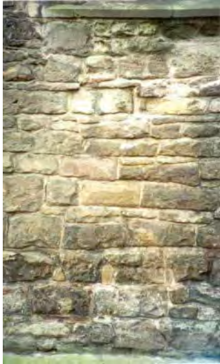
Figure 26. Mediaeval walling, St. Peter's Church: rough shaped Old Red Sandstone blocks with substantial mortared joints
