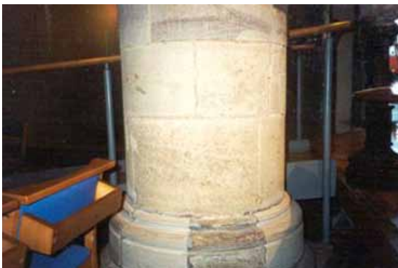
Figure 10. A pillar in the nave of All Saints Church. Lack of exposure to city fumes and possibly centuries of scrubbing has left the Old Red Sandstone almost white, though patches of reddish colour can be seen.
