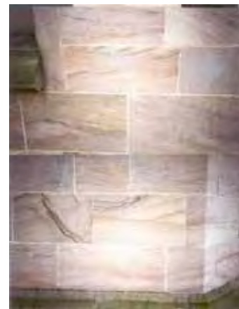
Figure 71. Sedimentary structures in the sandstone front of the New Library. The black lines are a later staining by circulating water after burial. The primary structures, cross- and graded-bedding, were likely formed in a delta.
